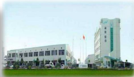
Commercial pump factory
